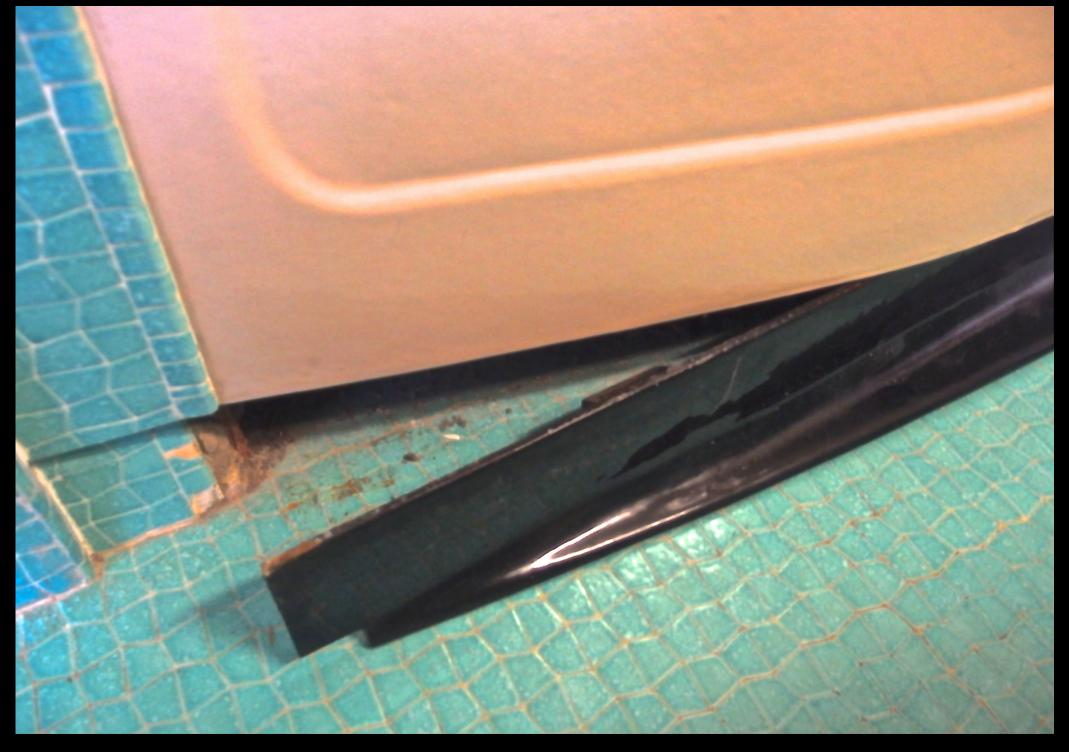
Removeable bathtub panel for plumbing repairs.
