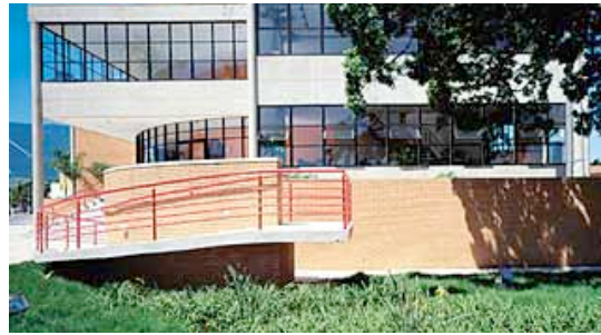
Façade in two angles: escadariae ramp for the disabled
