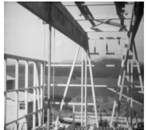
(2) Berta Rahm, Barn during construction, Nägelseehof Farm, Hallau, 1951
